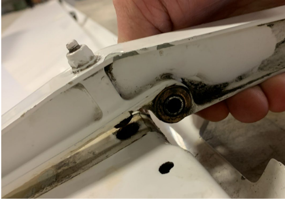
Figure 2 – View of removed elevator (upside down). Forward attachment bolt worn through lower skin.
