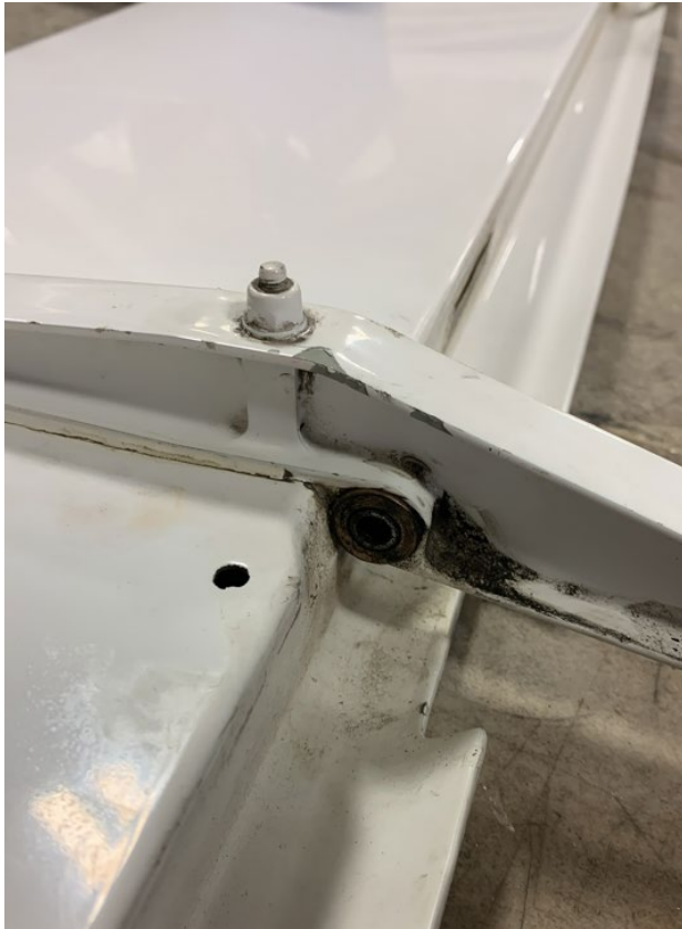
Figure 1 – View of removed elevator (upside down). Elevator control horn as installed on elevator.
