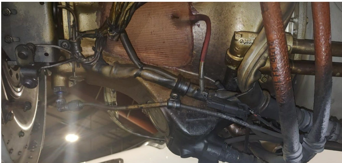
Picture 1 – Soot, signs of exhaust gas leakage
