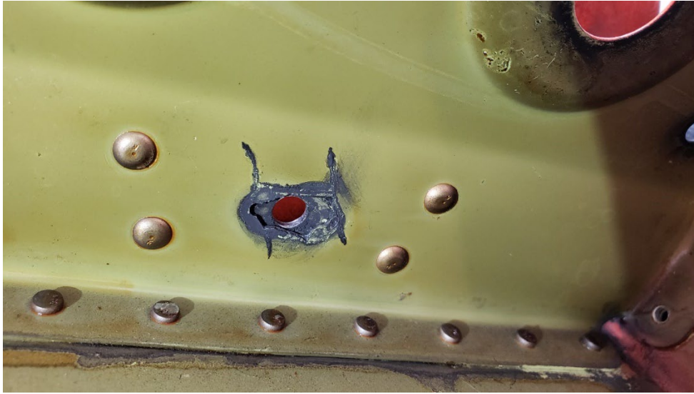
Picture 2 – Underside of rudder rib 6 with missing anchor nut
